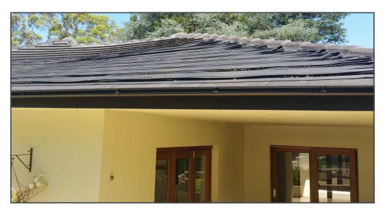
FTS was commissioned to investigate the cause and recommend remedial works by the local council to fix the roof failure of this luxury home in Pymble. Roof, beam hanging beams, strutting beams, underpurlins and some struts were poorly situated causing dislocation, slippage and rotation of beams.
