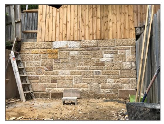
FTS provided full engineering design and slope stability assessment and site inspections during construction for the retaining wall which had failed in this heritage precinct of Paddington. Original wall photo below with a 150 mm lean forward at the top. Upon excavation it was found that there was no footing or wall thickening. The only access to build the wall was by hand through the rear Im wide ally.
