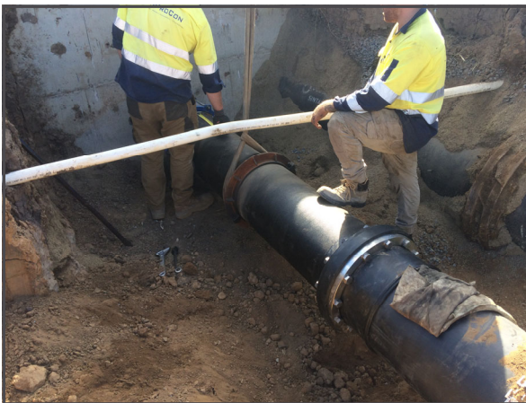
Valve chambers and associated flange fittings.
