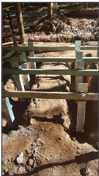
Basecourse, reinforcing, foundations for seats and picnic tables being set up within main shelter.
