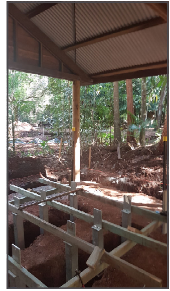
Basecourse, reinforcing, foundations for seats and picnic tables being set up within main shelter.
