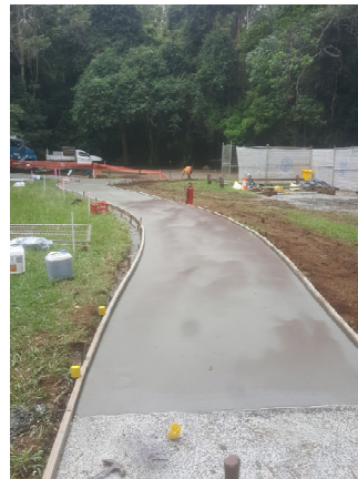
Concreting pathways, expansion and contraction joints, with washed aggregate finish
