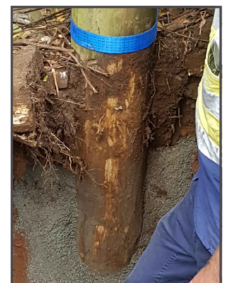
The left post was replaced and the other posts tested. Quality test samples from forensic investigation of the post timbers.
