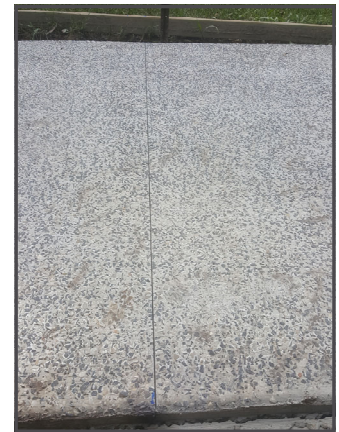
Concreting pathways, expansion and contraction joints, with washed aggregate finish
