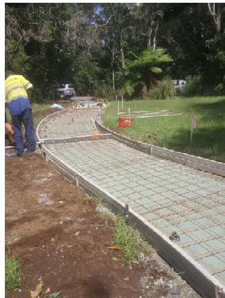
Concreting pathways, expansion and contraction joints, with washed aggregate finish
