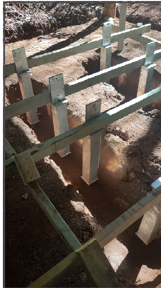
Basecourse, reinforcing, foundations for seats and picnic tables being set up within main shelter.
