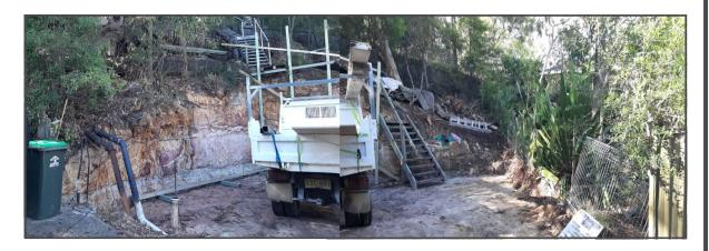
FTS organized to have the exposed rock and services assessed by JK Geotechnics following the exposure of a remnant clay seam within the rock layers.
