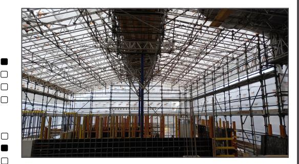
Engineering design certification of temporary roof shelter system using Kwikstage scaffold components and tubing to AS1576 with Monarflex Airflow 166gsm reinforced LDPE roof sheeting.
