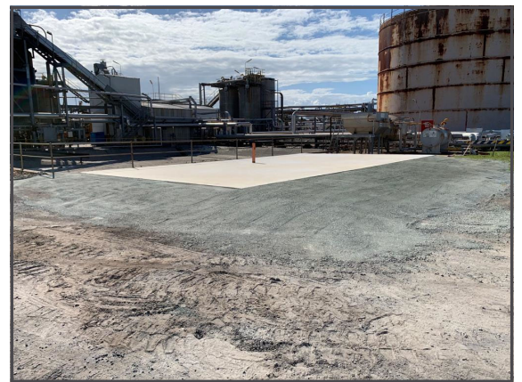
Base ballast preparation, form, reinforcement placement and place concrete.
