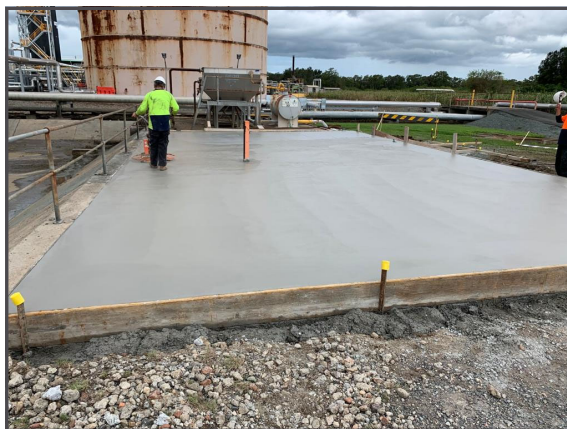
Base ballast preparation, form, reinforcement placement and place concrete.
