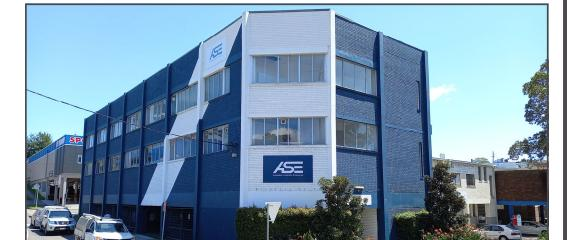
FTS was commissioned to assess the floor load capacity for a reinforced concrete building without asbuilt or design drawings being available. This was undertaken using a hand held radar device that could determine bar size, depth and alignment, to survey the reinforcement and a Schmidt Hammer to indicate concrete strength.. ASE were installing a new 3T freeze drier on the first floor.
